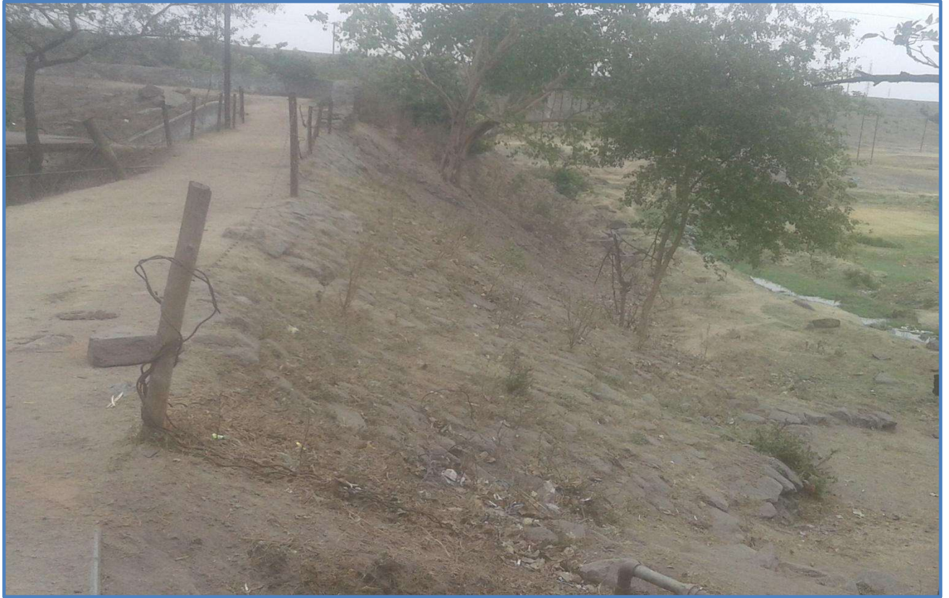
Picture 3 - Stone Pitching/embankment at Kari Jore
