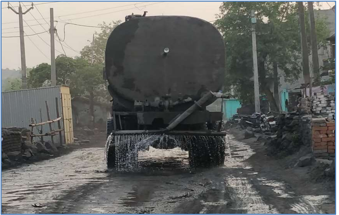
Picture 2 – Water Sprinkling on Transportation Road
