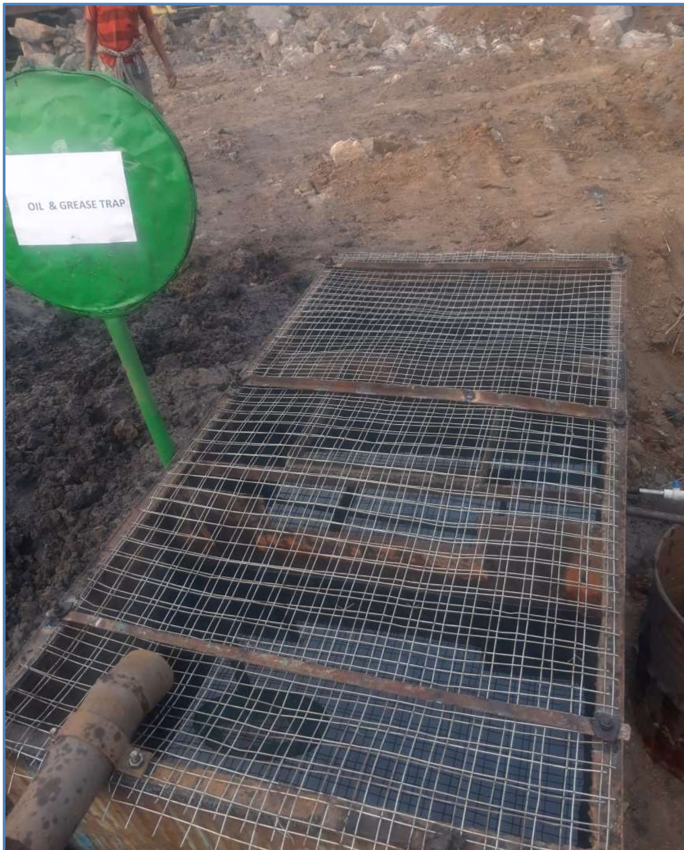
Picture 5 – Oil & Grease Trap
